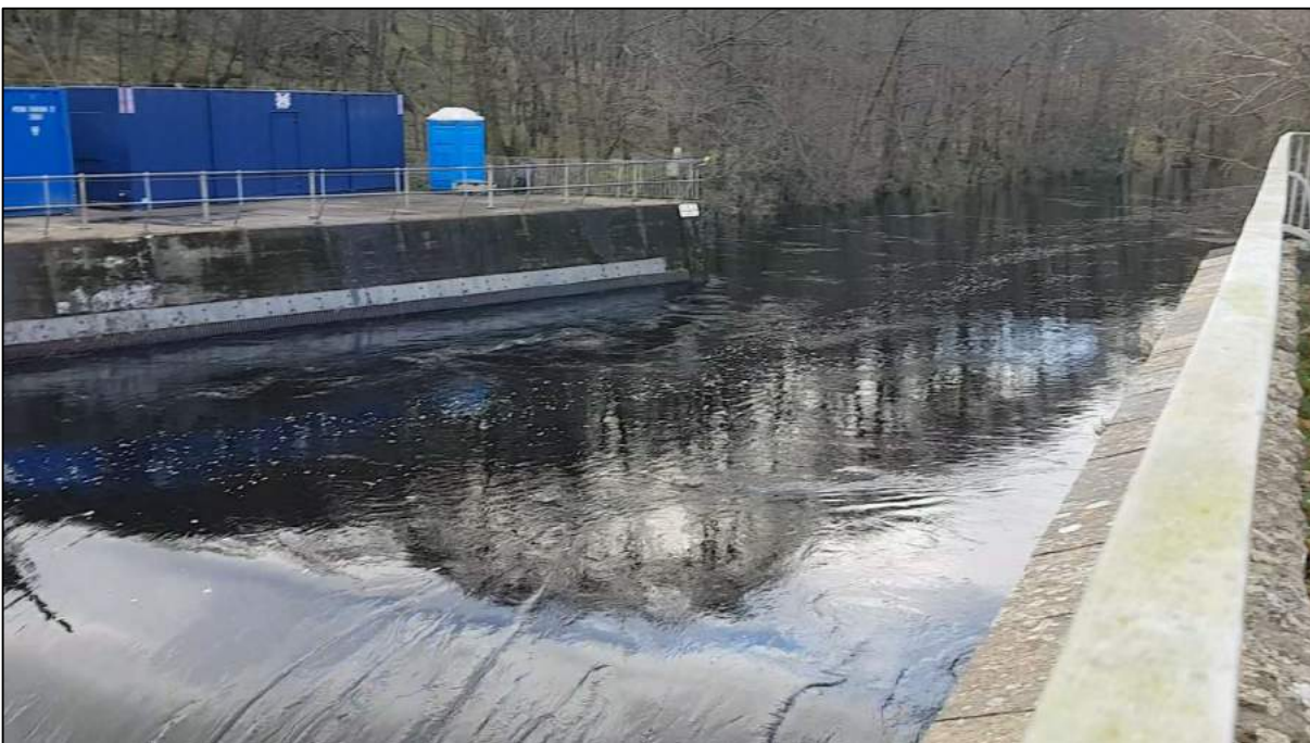
Photograph 2 - Looking upstream from hydro weir towards the stretch of the river downstream of the site. On the left is the intake grill for the tunnel to Dalchonzie power station.
