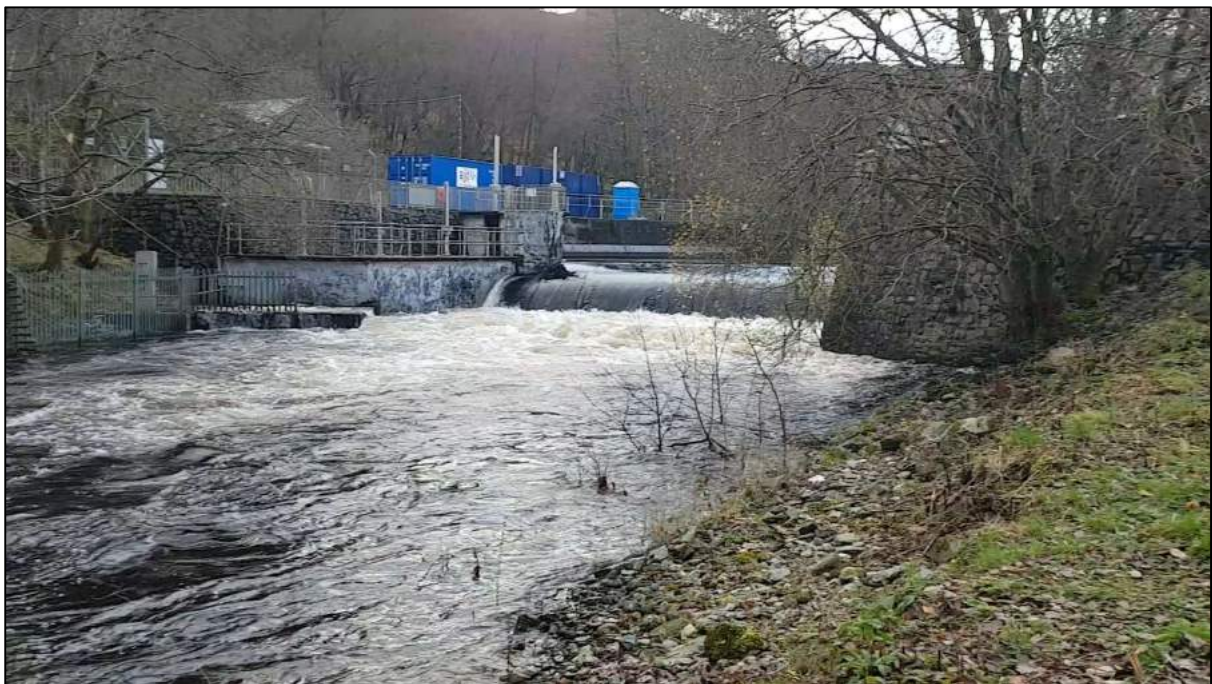
Photograph 4 - View from downstream at the SSE hydro intake and weir (on left of picture) and retaining wall on right (at street level of main road through St Fillans). On the left of the weir there is the outlet from the fish pass.
