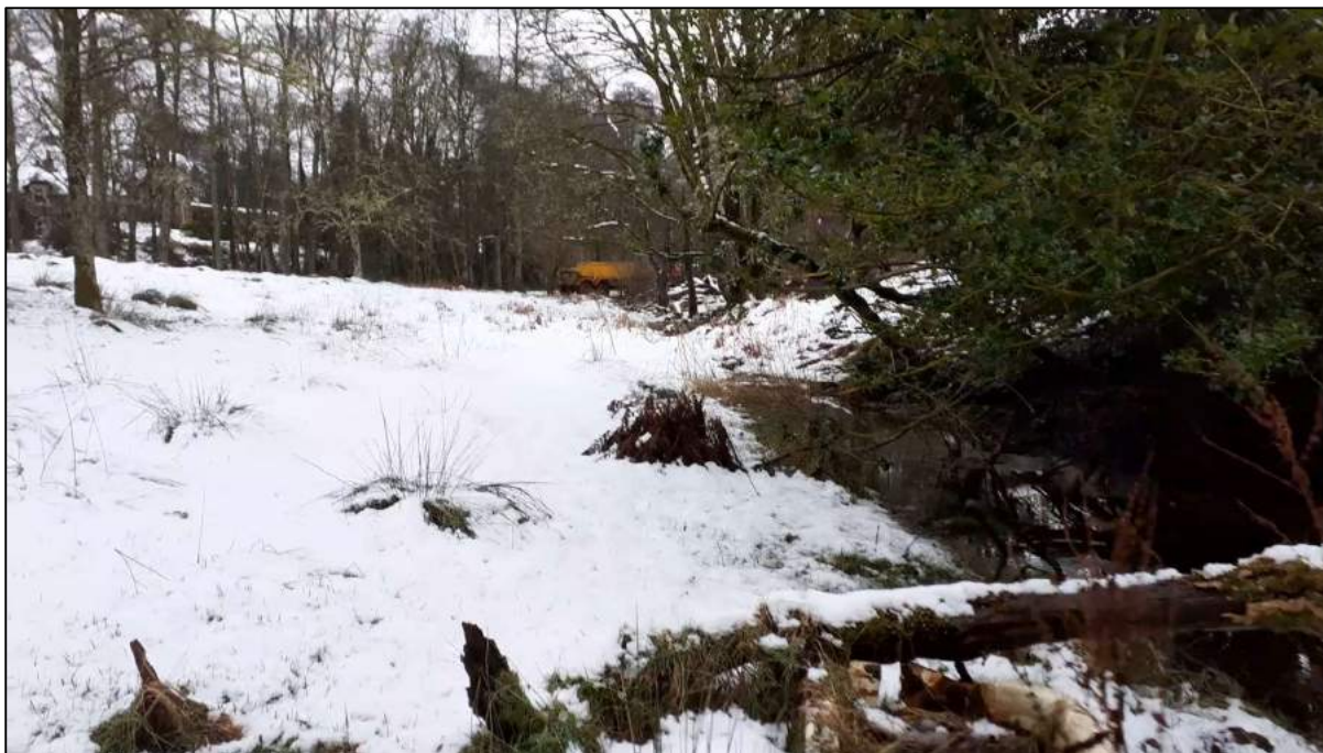
Photograph 15 - Looking east along line of “flood relief channel”. The vehicle in the distance is sitting roughly on top of the culvert where the field entrance is situated. The culvert discharges onto the bank of the River Earn just beyond.
