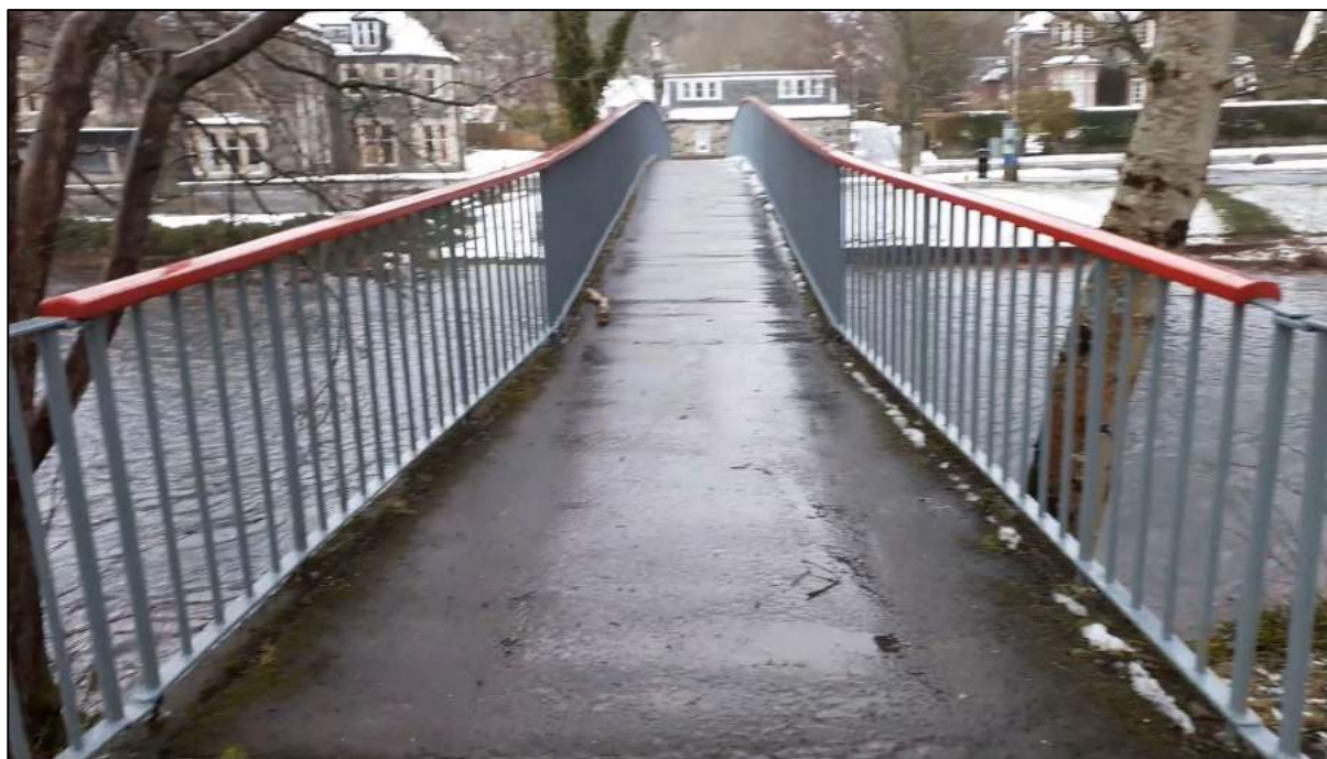
Photograph 7 - View north across the footbridge towards the main road (A85) and houses in St Fillans
