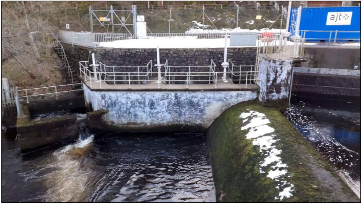
Photograph 3 - River Earn flowing over hydro weir, with intake screen to tunnel and fish pass structure on opposite bank.
