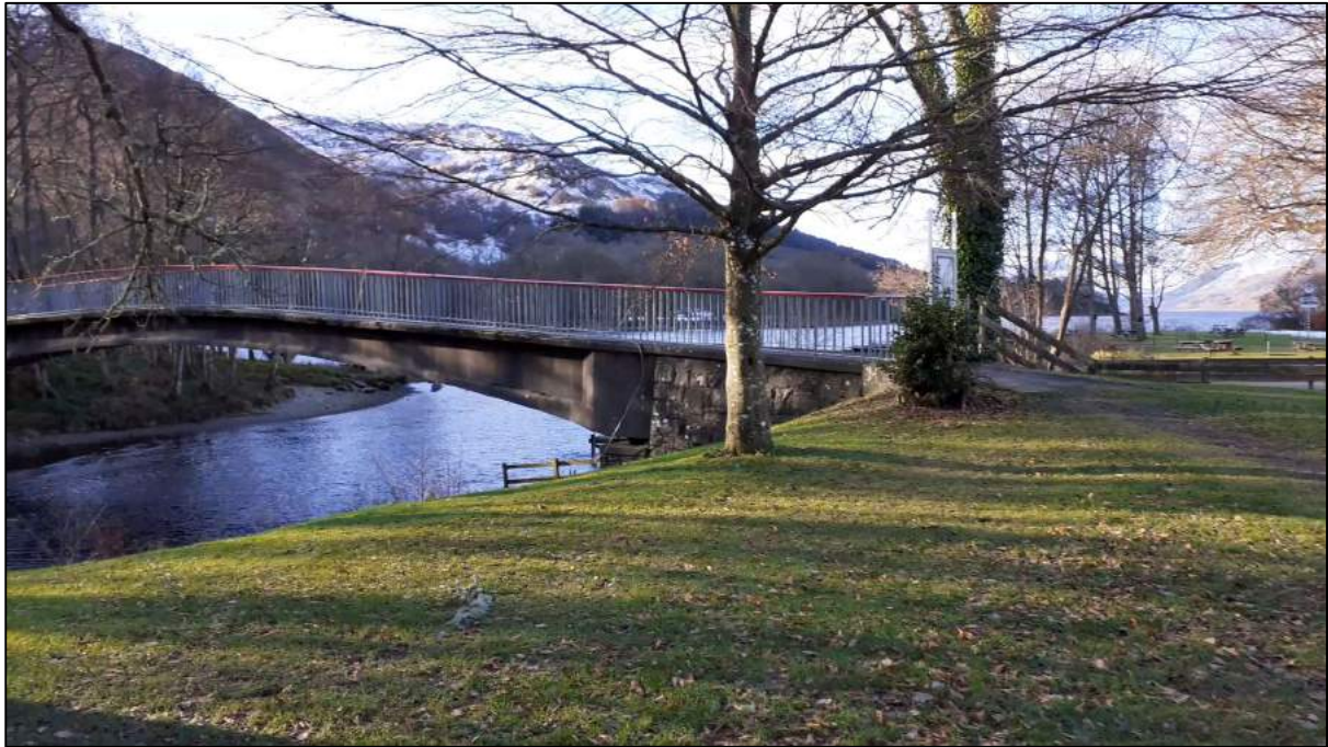
Photograph 5 - Looking upstream along the River Earn past the substantial footbridge near the upstream end of the river. A short distance upstream, Loch Earn is visible. On the opposite bank the landfall of the bridge is on the north west corner of the site.
