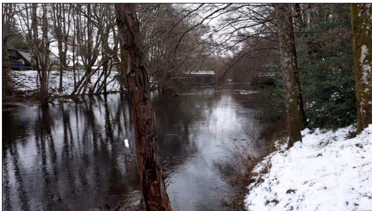
Photograph 17 - From the right bank to the River Earn, at the eastern corner of the site, looking towards the hydro weir which is approximately 100m downstream.
