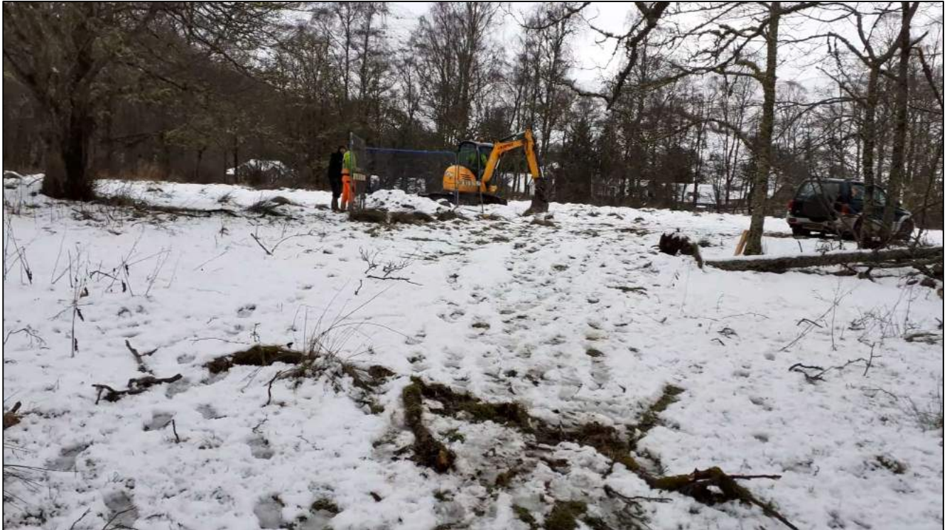
Photograph 3 – Looking north to centre of site, with drainage testing underway in TP1. The high point of the site is immediately behind (recommended location for main building)
