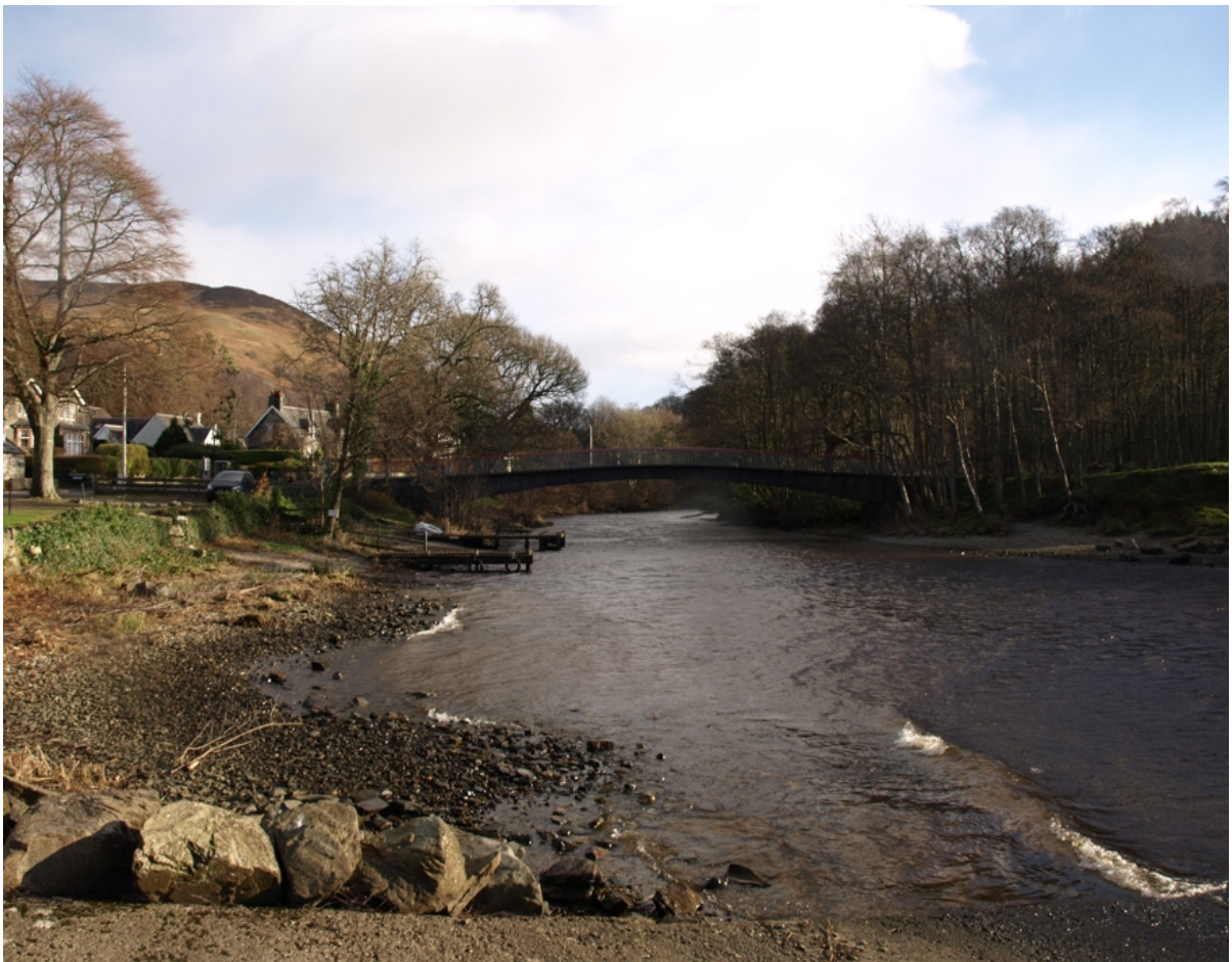
Footbridge 2 over River Earn to site. For Saint Fillans Community Council
