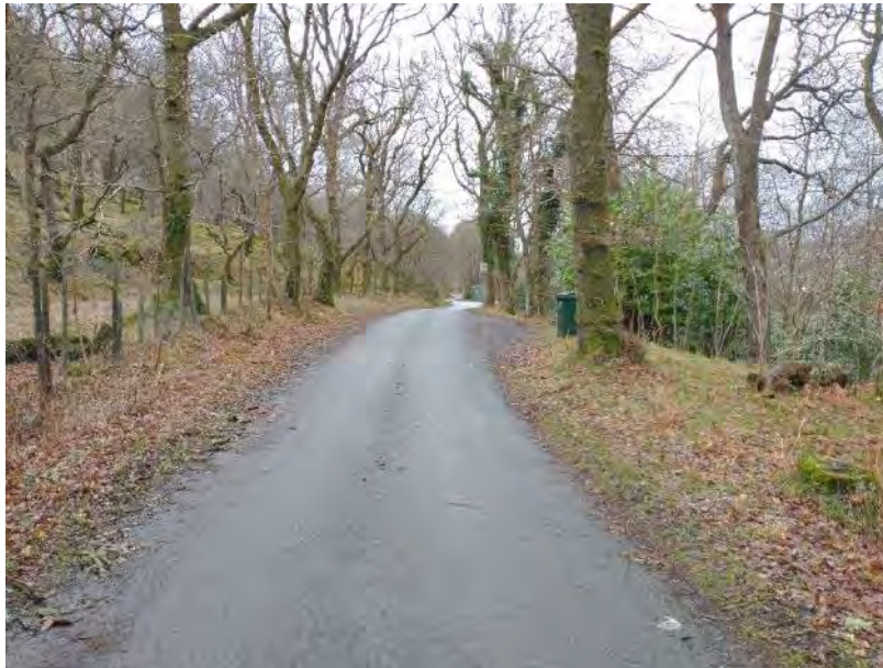
Figure 2-2 - South Loch Earn Road showing passing place
