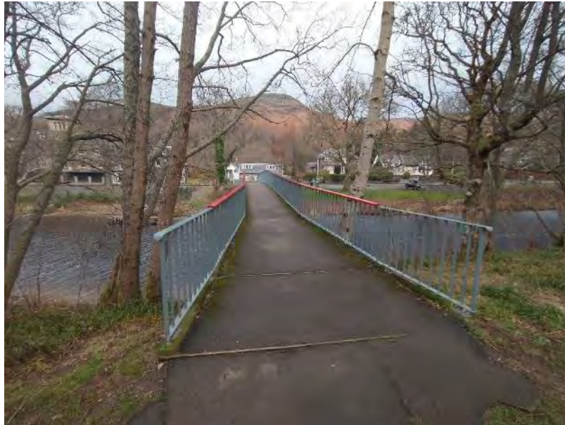
Figure 2-5 - Bridge across the River Earn
