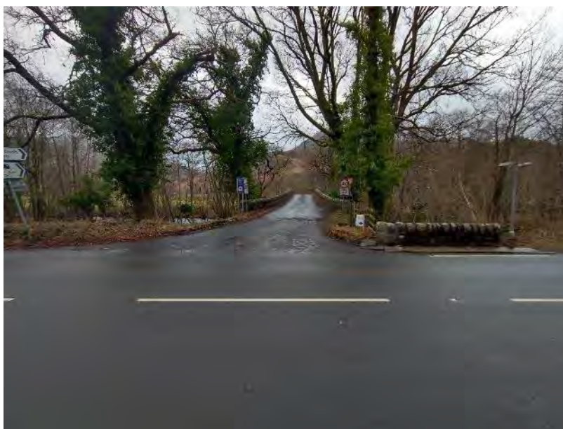
Figure 2-1 - Existing access on A85 to South Loch Earn Road
