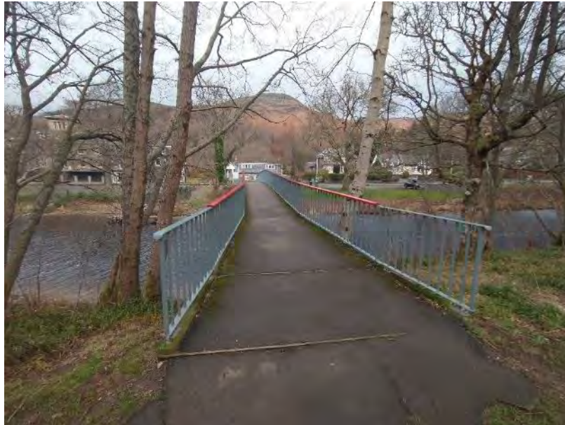
Figure 2-5 - Bridge across the River Earn
